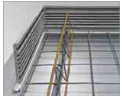
Permanent edging formwork made of fibre-reinforced concrete
