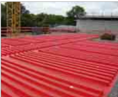
Administrative building, Munich (Germany) Fratec formwork
