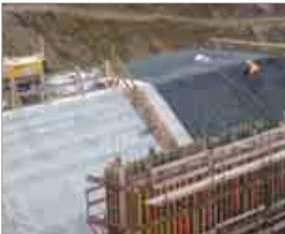
Finnetunnel, railway line Erfurt - Leipzig/Halle (Germany) Spacers made of fibre-reinforced concrete, Zemdrain® formwork liner, Stremaform® formwork elements
